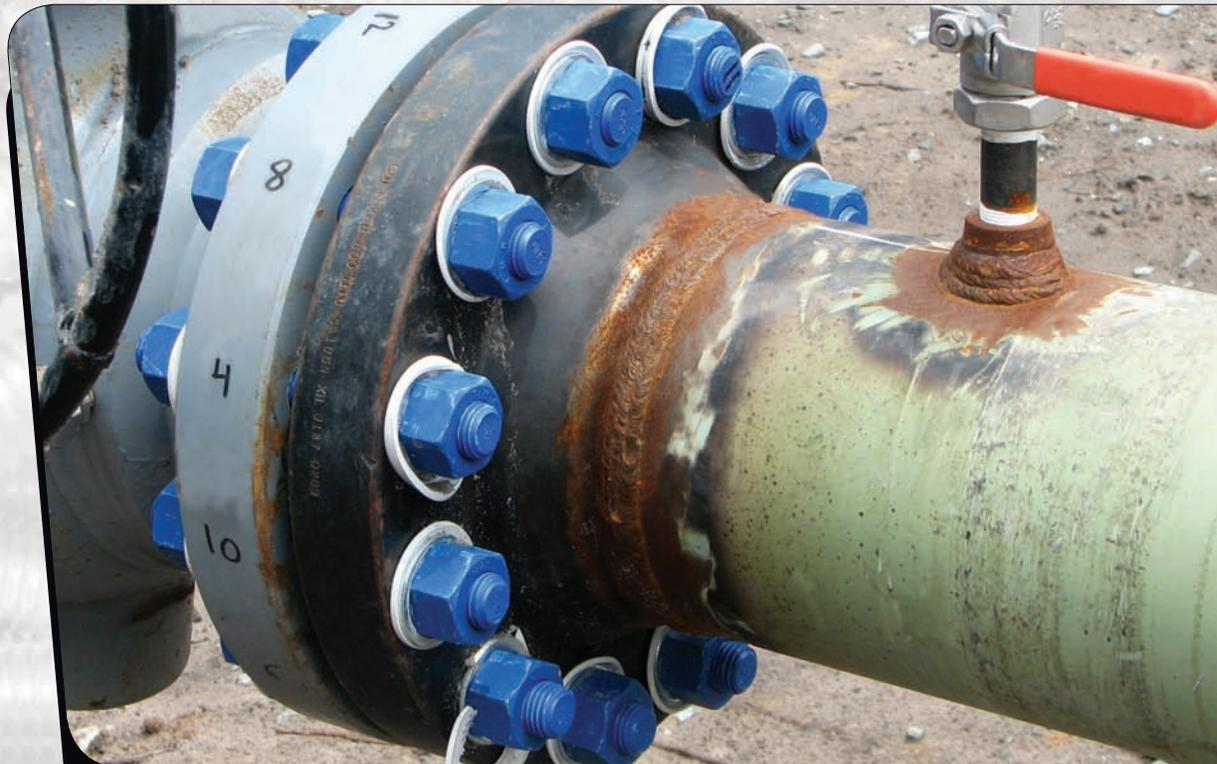
*There is concern of extrusion and cracking of insulation kit sleeve and washer assemblies in high-torque applications*
